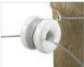
**Round Donut With Wire** The line for this type of phone service was usually on porcelain insulators called “donuts” which are hung from a tree with telephone wire running through the hole. You can still find telephone hexagon donut insulators on trees along Hugo Road.
